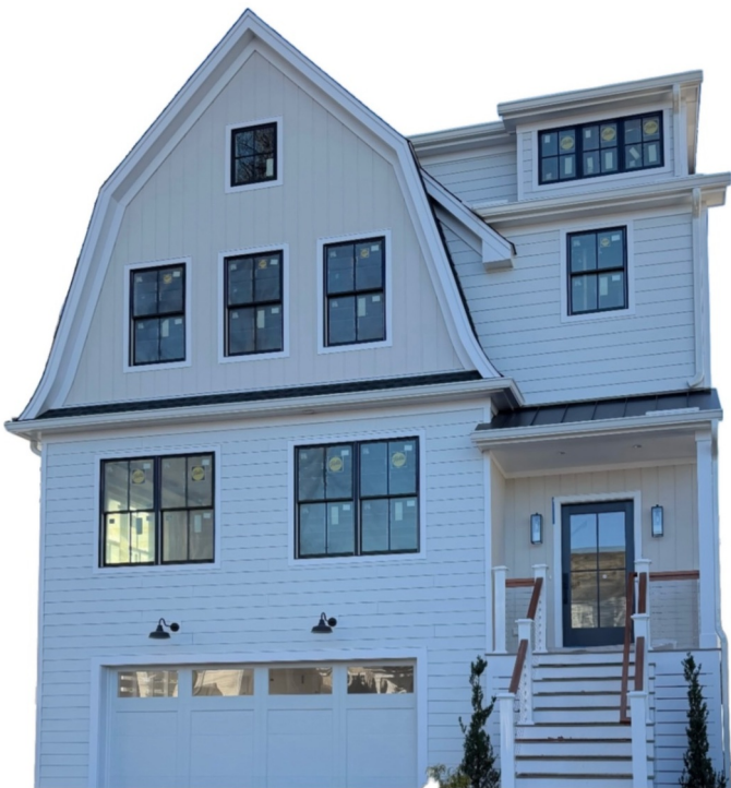
A Green Atlantic PVC job — specialty trim at every window and door, with our trim, corners and soffit throughout.
