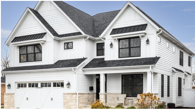
Water table set below the first course, with our trim and corners above.
